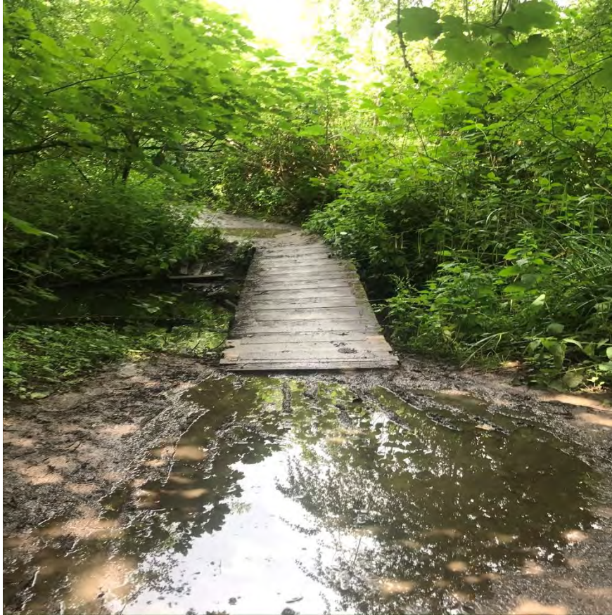
Figure 4: Footpath leading past the Crowne Plaza, connecting the Thames Path with the area around Westhorpe House (location 7 in table). This view northward shows parts of the muddy track, an old slippery footbridge and overgrowth.
